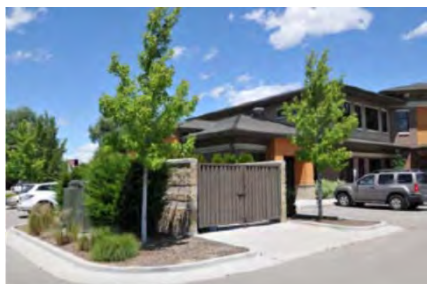
Well-designed service enclosure example.
